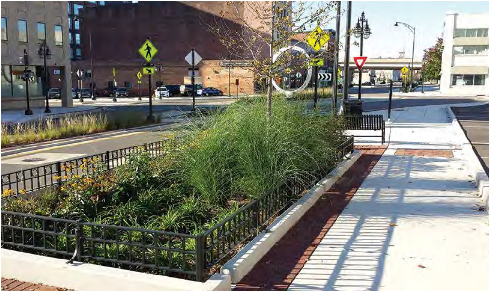
Figure 42: Bio-Based Stormwater Infrastructure (Bioswales) in Downtown Peoria
