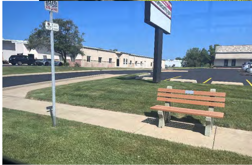
Figure 135: Two Examples of Existing Bus Stop Infrastructure
